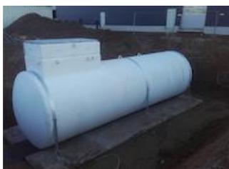
Process oil is stored in an underground tank (Fig. 04). A desired dosage travels now through the pipelines into the mixing vessels. The tank equipment and the filling point have been designed and constructed fulfilling the requirements of the German Water Resources Law (WHG) and the Regulation on Facilities Handling Substances hazardous to Water (AwSV).
