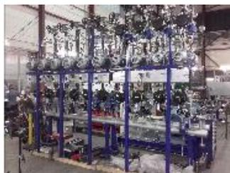
The temperature of the entire process is automatically controlled at the thermal oil secondary station (Fig. 02). The users have been combined according to functional affinity in separately regulated heating loops.
